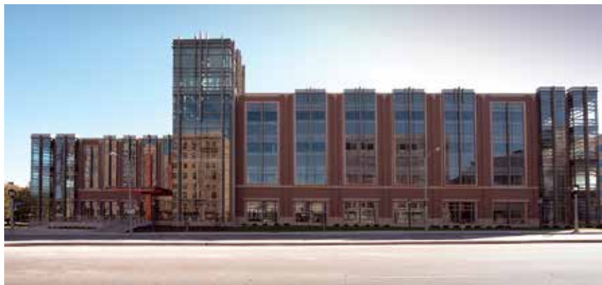
Marquette University's 115,000-square-foot College of Engineering building consolidates four engineering departments and includes lab space, offices, classrooms, and other needs. The building, which achieved LEED Silver certification, features architectural precast concrete panels embedded with half bricks and accented with cast-in, limestone-colored lintels and headers. All photos: HGA.
